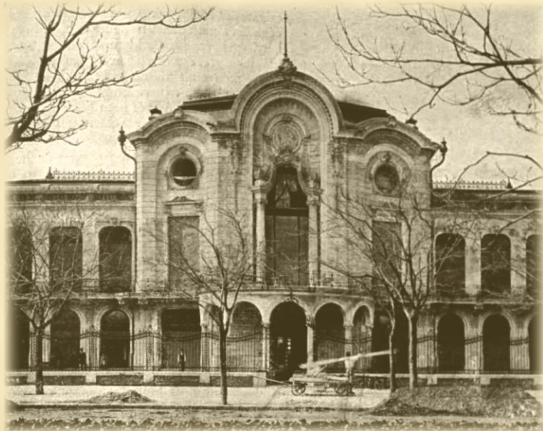
The palace under construction*
