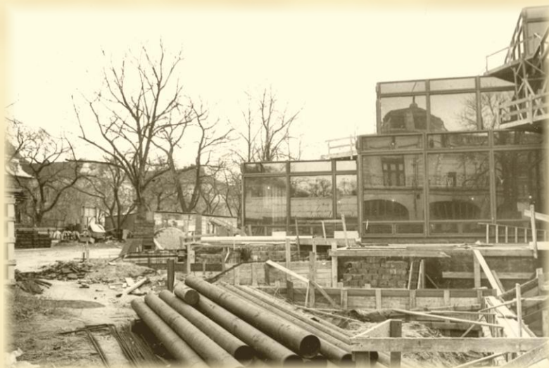
The cultural centre under construction*
